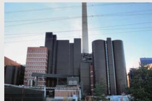
At Salmisaari B, the SCR system was installed in a pulverized coal fired boiler. Retrofitting a fully built environment with urea storage, hydrolysis equipment and a catalytic reactor was challenging. (Photo: Helen Ltd.)
