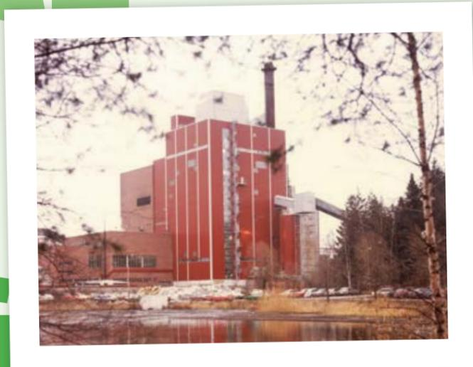
Commissioned in late 1984, a Valmet-delivered bubbling fluidized bed boiler (BFB) has been serving Stora Enso's fluting mill in Heinola, Finland, for nearly 250,000 hours.
